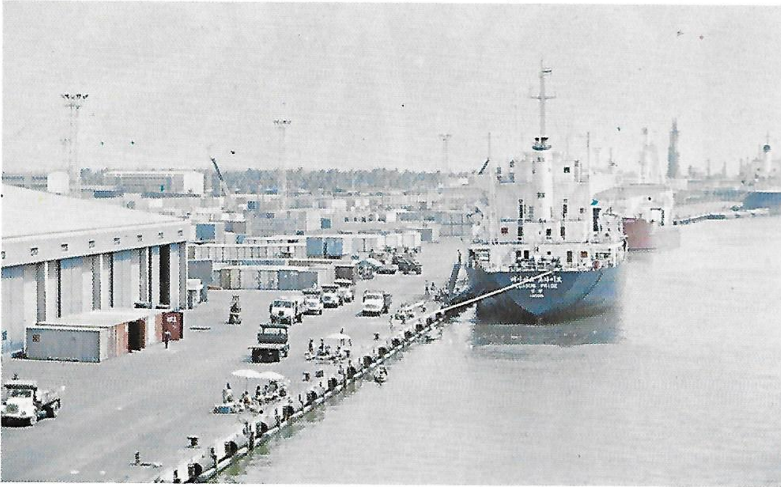
A view of the container berth at Bangkok with "Pegasus Pride" in the foreground.
