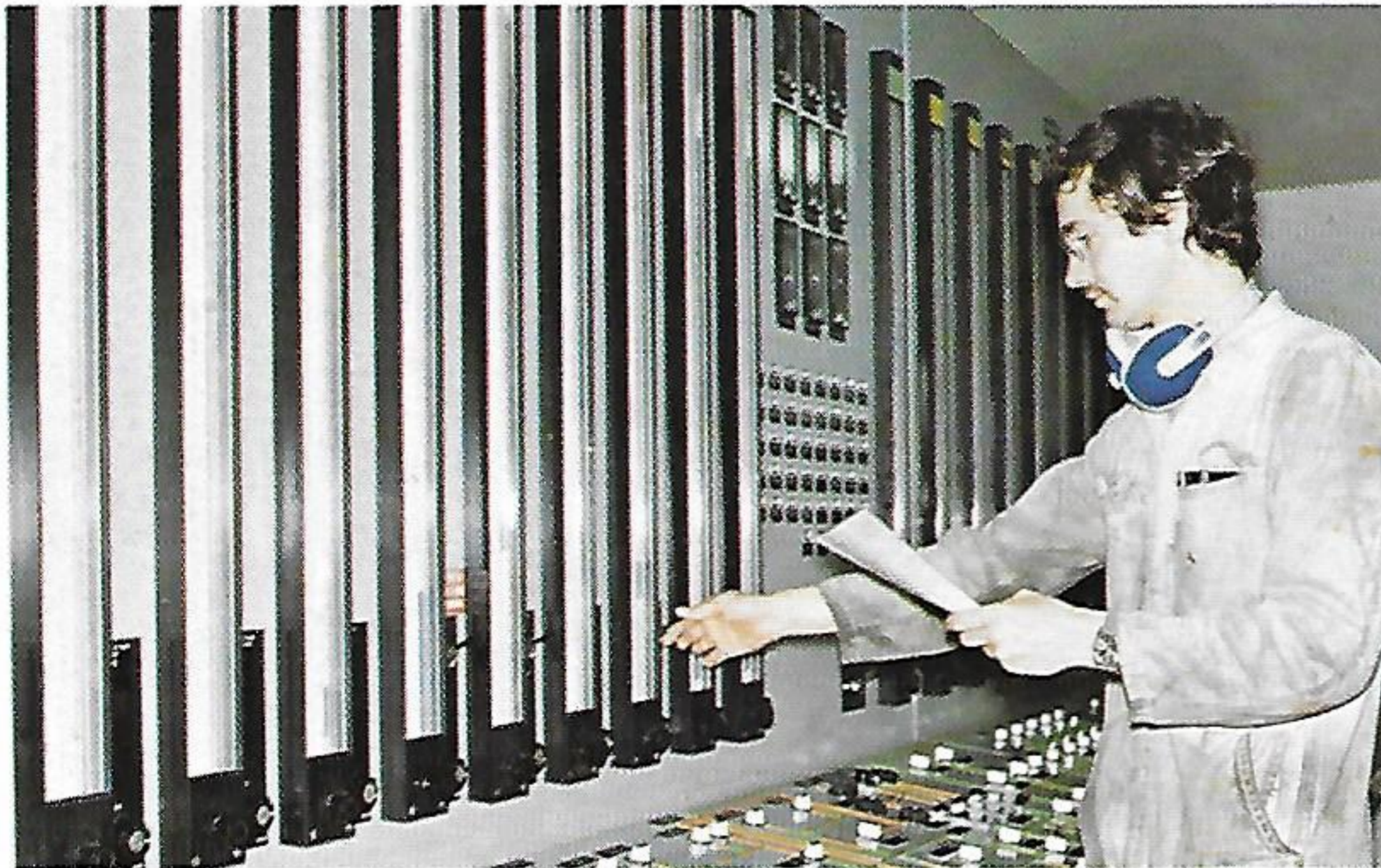
Gauge glasses are checked to see that the ship is properly trimmed by Senior Third Engineer William Carson.
