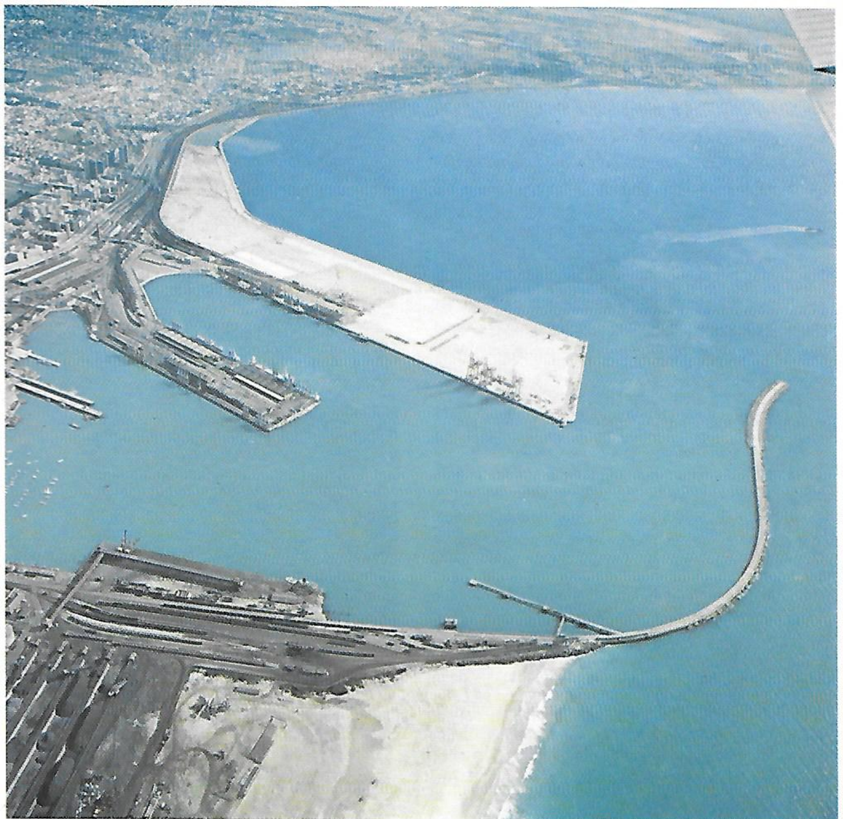
Work on the expansion of Port Elizabeth Harbour is nearing completion. The widened Charl Malan quay is pictured and the extended breakwater can be seen at the right of picture.
