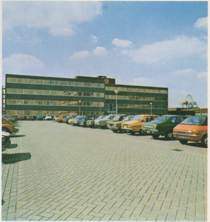
Conva's modern offices strategically located close to a motorway and the Rotterdam Container Port.
