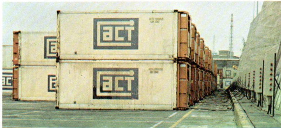
Partial view of the new refrigeration facilities which include 40 pillars with a capacity for 240 20-foot reefer boxes stacked in bays two high and three rows deep.
