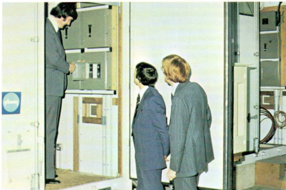
Partial view of the inside of the specially adapted container for the Plessey Pentex electronic telephone exchange shipped to Transkei. Explaining how the exchange functions is Mr. Dick Riley (inside container), Plessey's Regional Contracts Manager for the Electronic Exchanges Division, to Mr. Tom Roddis, EHCL North Midlands Sales Representative, and Mr. Barry Thorley (right), Plessey's Shipping Manager for Beeston.
