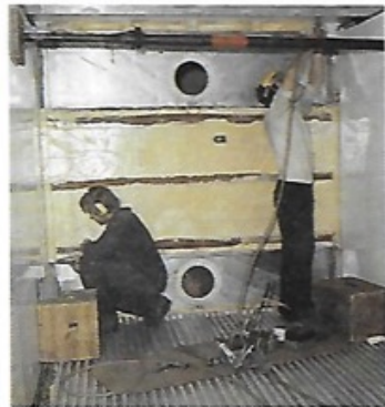
The recycling of 1,250 refrigerated ACT containers to improve thermal efficiency is taking place at Concargo's plant at Weston-super-Mare. The containers are stripped down completely and then rebuilt. In the photographs (left to right) the flooring rails are laid; polyurethane foam for insulation is press-injected in panels; the components are riveted; the inspection of newly recycled container is carried out by Mr. Bernard Glynn (left), ACT Services' Container and Equipment Inspector in charge of approving the completed work, and Mr. Alan Hollier, Estimator, of Concargo.
