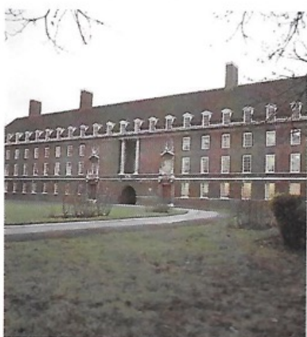
The 110-bedroom Nurses Home is located just across the street from the hospital.
