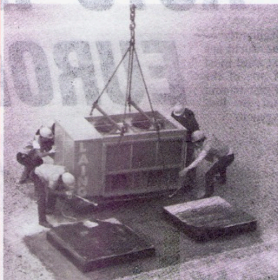
Releasing the new air-conditioning equipment from its harness
