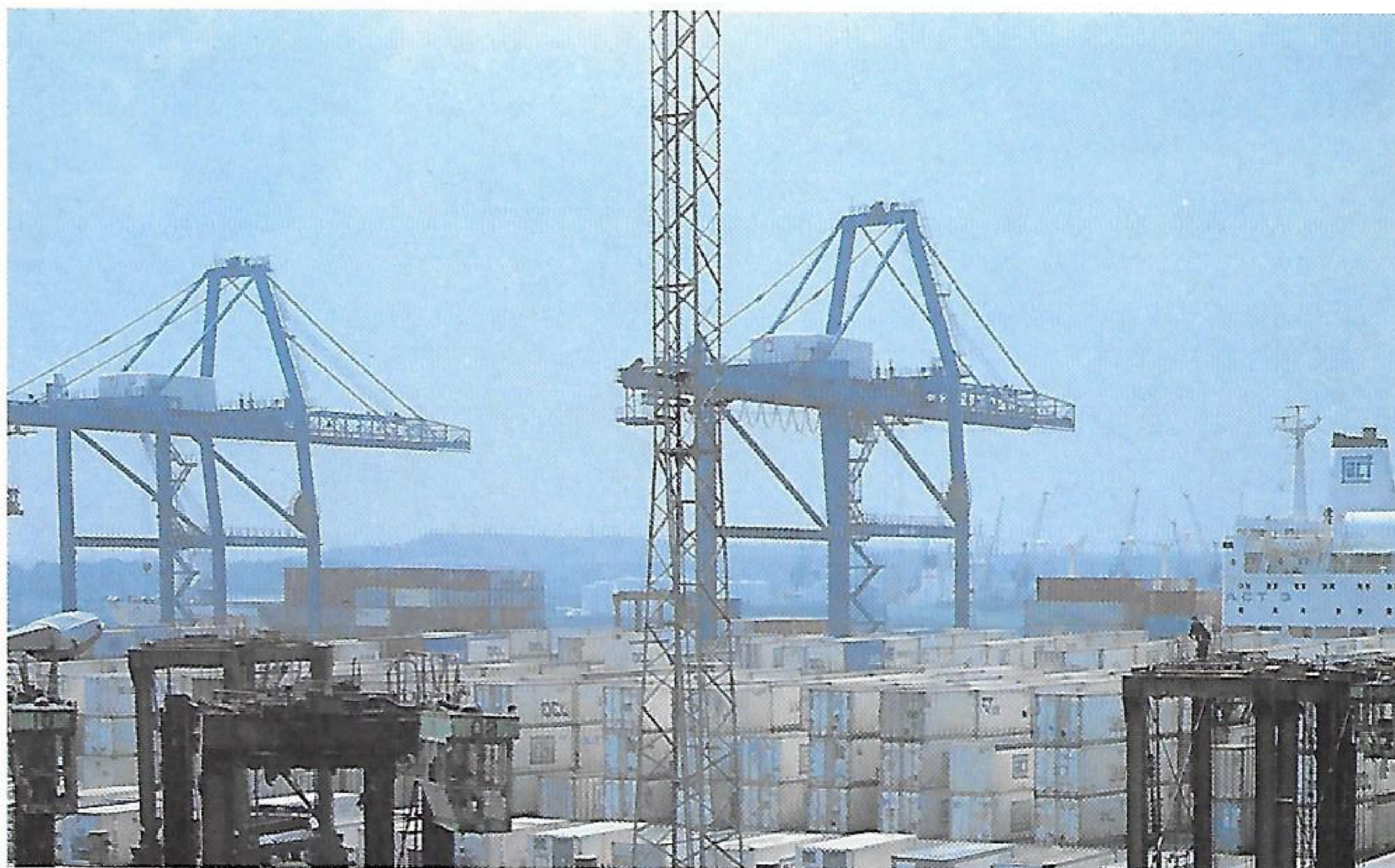
Partial view of Northfleet Hope looking towards the riverside berth.
