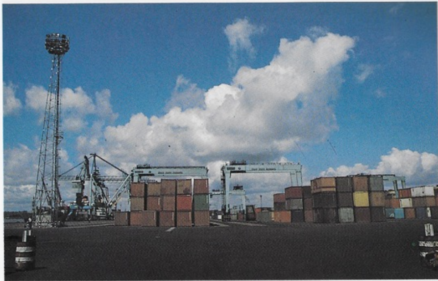
Yard gantries at work at the Container Terminal, capable of handling 250,000 20-foot equivalent units per year.
