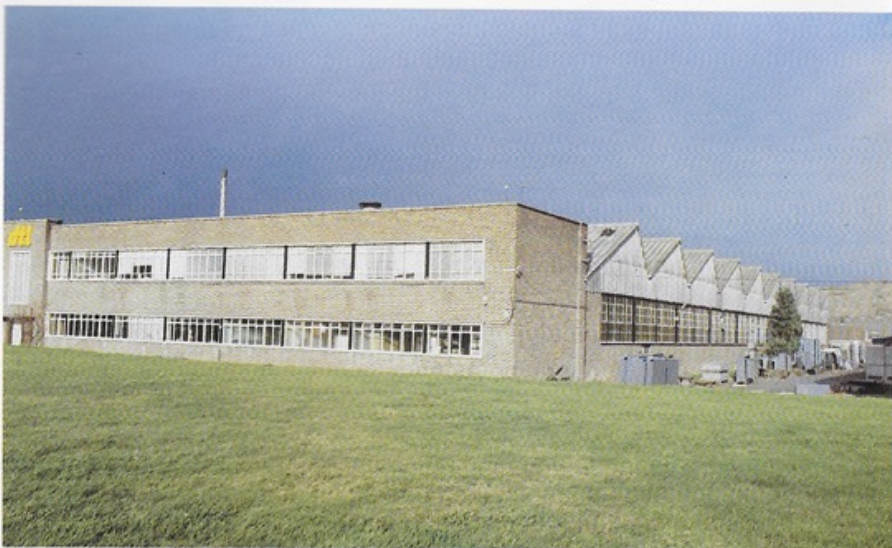
Partial view of Peebles Distribution Transformers' modern, purpose-built factory at Broxburn in West Lothian, where a broad range of transformers are produced for rural, urban and industrial systems as well as for the mining and oil industries.
