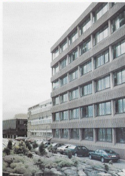
Partial view of Allied Colloids' Low Moor premises at Bradford, showing sales and administrative offices and research block.
