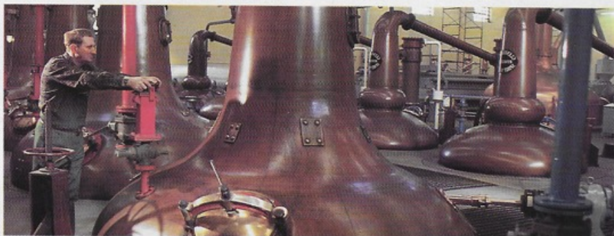
Partial view of the Stillhouse at the Glenfiddich Distillery of William Grant and Sons. Glenfiddich is distilled twice in traditionally shaped copper stills built and maintained by the Company's own coppersmiths.
