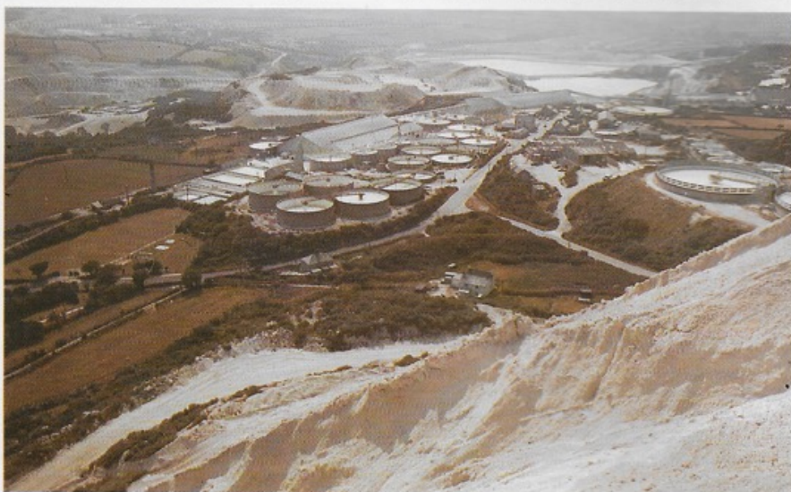
Partial view of a production complex for English China Clays near St. Austell in Cornwall.
