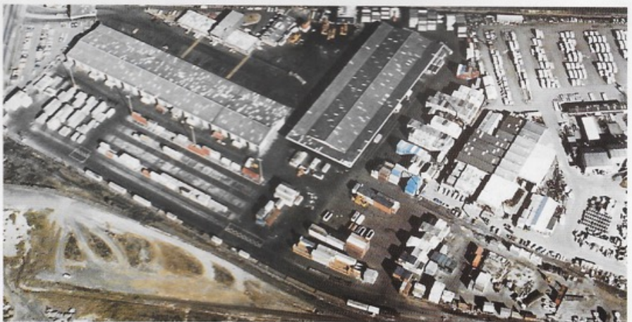
At the other end of the line, ACT(A) has increased its share in Liner Freight Services, Sydney, and the 20-acre site in the centre of the large industrial area of South-West Sydney (pictured) has a working capacity of 1,500 containers with mobile equipment enabling rapid movement and stacking. Facilities are available for both the cleaning and repair of containers on site. The complex is linked by rail to the Glebe Island Terminal in Port Jackson and the Terminals in Botany Bay. There is excellent road access and three rail sidings link the depot with Sydney's major city and country lines.
