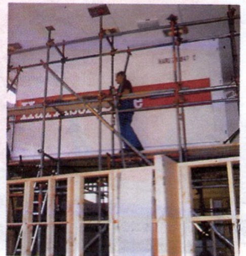
After gently being lowered onto metal "rollers" (photo at left) the container is eased inch-by-inch through the frames from which the windows had been removed (photo at right).
