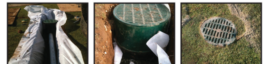
Photos from a typical 12" round catch basin installation.
