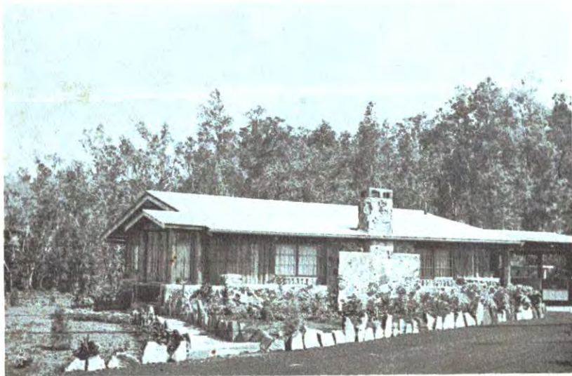
Home of Mr. and Mrs. Joe Fergerstrom after they completed planting their lawn and landscaping. Their attractive home is constructed of materials found on the subdivision, Ohia wood and native stone.
