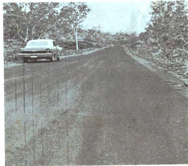
One of the 120 miles of excellent streets completed within the subdivision.
