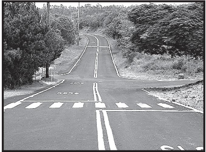
The road past Kabuku Park, with new crosswalk markings, signage and reduced speed limit, as well as a couple of speed bumps to control traffic.
