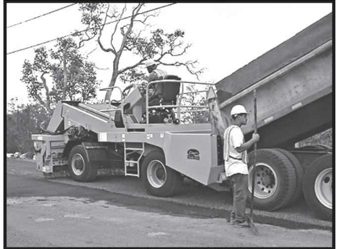
*Connecting the two big machines ensures a smooth flow of chip into the spreader hopper, and eliminates the dangers of trying to keep them together*
