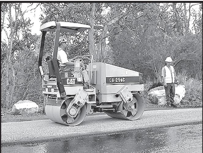
*Rolling the fresh chip into the oil makes the surface flatter, harder and more stable.*
