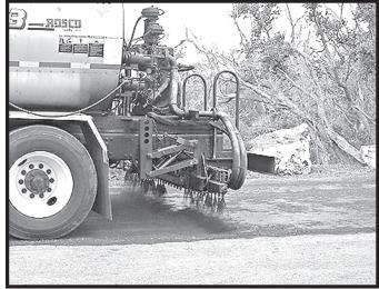
Once the surface has been prepared, the oil truck spreads a layer of specially-compounded road oil
