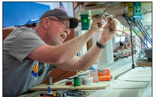
Craig Faris installs wiring under the layout
