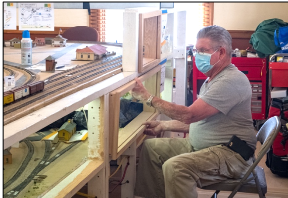
Ken Nelson installs a window into the lower Level benchwork. The oak materials which match the museum building trim were donated to ARHS by Spellman Hardwoods of Phoenix.
