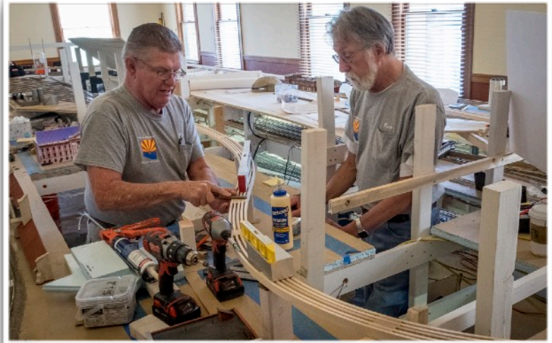
Ken Nelson and Ken Wolfe check the grade on the spline sub-roadbed connecting Mobest yard to Prescott.
