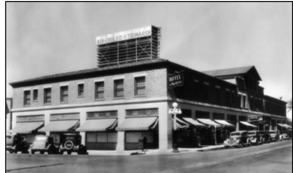
The Rebuilt Hotel Congress Tucson fire foundation photo
