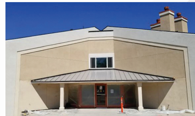
Katherine Bates Apartments - Entrance (After)
