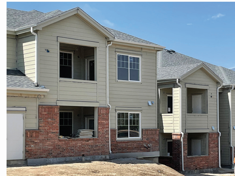
Shooks Run - Street View (Construction Phase)
