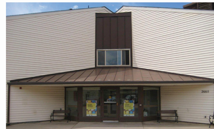
Katherine Bates Apartments - Entrance (Before)
