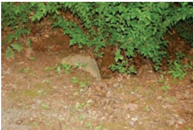
Figure 13. Pipe under the gravel access road. The associated ditch requires maintenance and the crossing should be marked.
