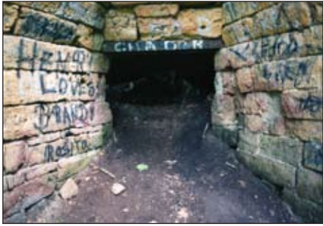
Vandalism evident at Bourbon Furnace, part of the Bourbon Iron Works (KY1000), Bath County, Kentucky. Photo by David McBride.
