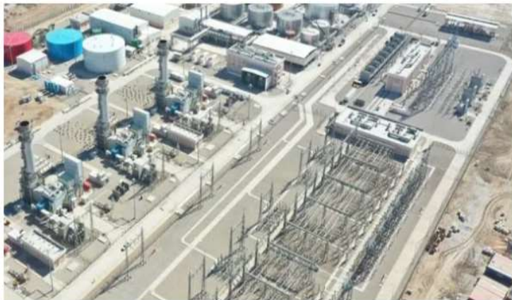
SAMAWA Combined Circulation Power Plant
