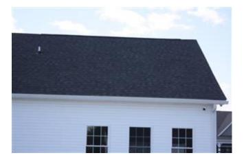
**Gutters and Downspouts.** The buildings have aluminum gutters and downspouts. The gutters and downspouts are in good condition.
