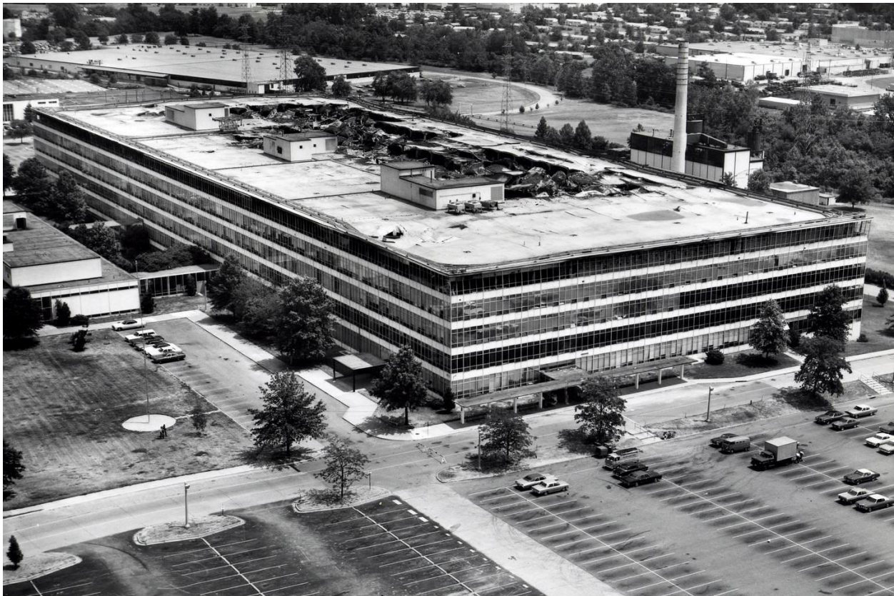
This photo provided by the National Archives and Records Administration shows the damaged sixth floor and roof of the Military Personnel Records Center in Overland, Mo., near St. Louis, after a massive fire that started on July 12, 1973. (National Archives via AP)
