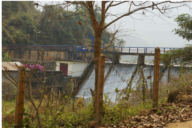
Figure 10. Hydroelectric power is produced from a small dam on a Mekong River tributary in northern Lao PDR highlands. The reservoir behind the dams is used as a fishery and for irrigation.
