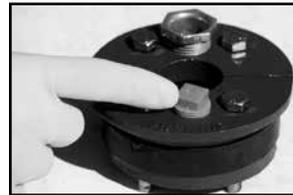
Some wells have a sanitary seal with either an air vent or a plug that can be removed (a).
