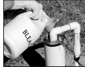
4. After the bleach has been added, run water from an outside hose into the well casing until you smell chlorine coming from the hose.
