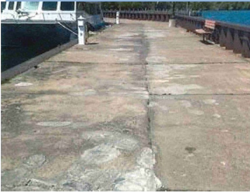
Concrete Spalling on the South Leg (source: City of Bayfield)
