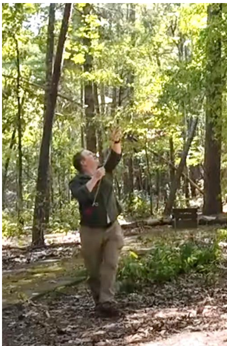
K4SWL throwing an arborist line over a tree branch for an endfed antenna.
