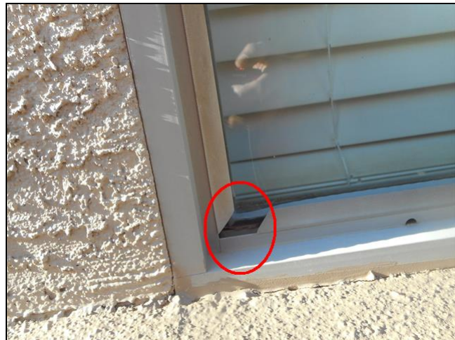
2.2 Item 4(Picture) Master bath exterior window
