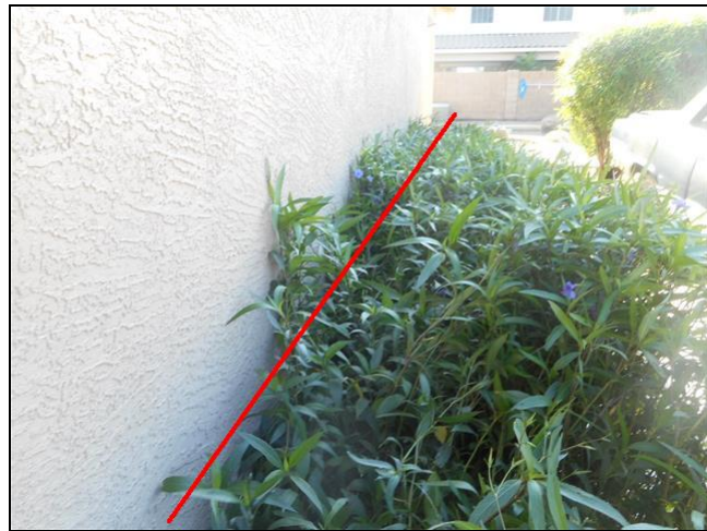
2.4 Item 2(Picture) North side exterior wall
