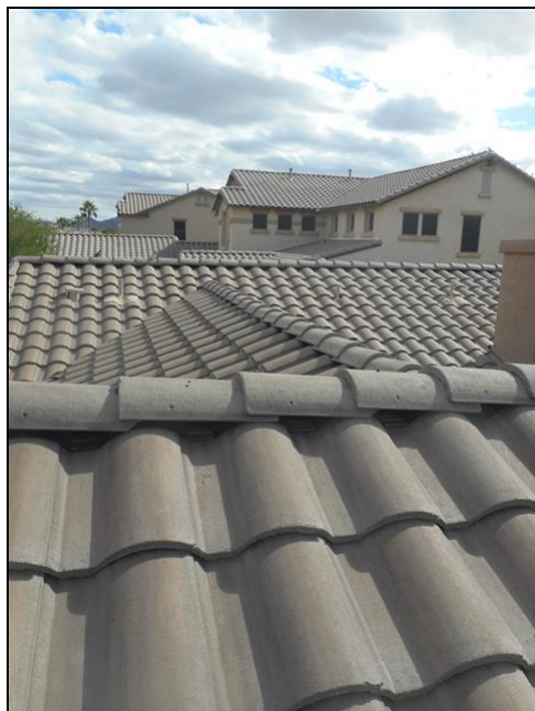
General shot of roofing (pic 3)
