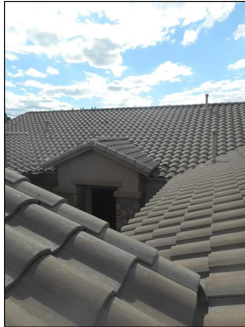
General shot of roofing (pic 2)
