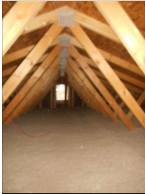
General shot of insulation in the attic
