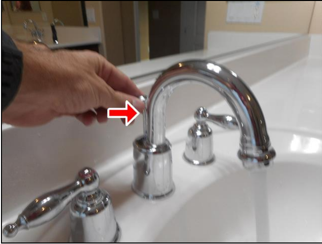
5.1 Item 2(Picture) Faucet next to bath tub
