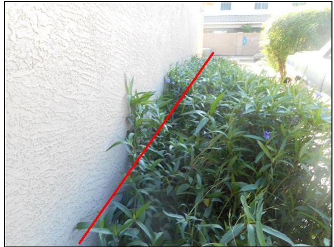
2.4 Item 2(Picture) North side exterior wall
