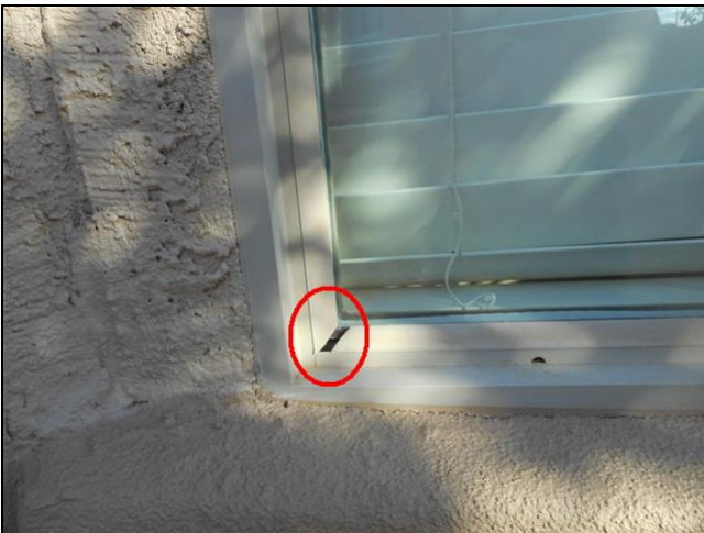
2.2 Item 3(Picture) Backyard window next to paver patio
