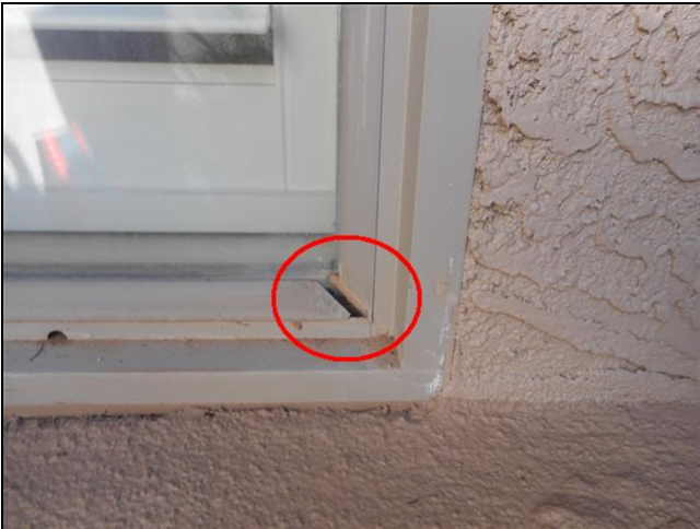
2.2 Item 1(Picture) Courtyard area
