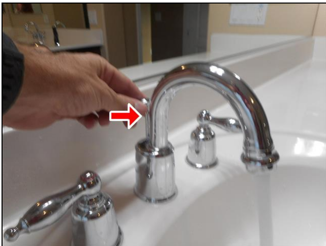
5.1 Item 2(Picture) Faucet next to bath tub
