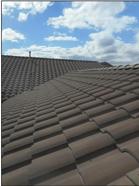
General shot of roofing (pic 1)
