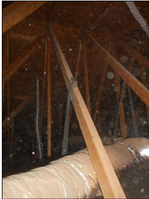
General shot of wood trusses and attic
