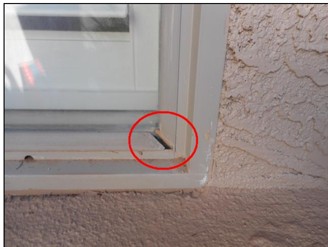
2.2 Item 1(Picture) Courtyard area
