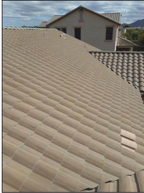
General shot of roofing (pic 5)
