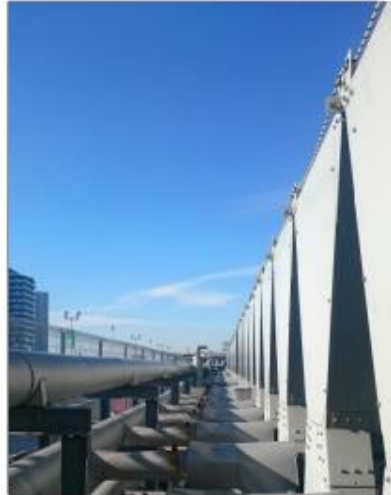
Heat pump condenser units (centralised & stand alone)
