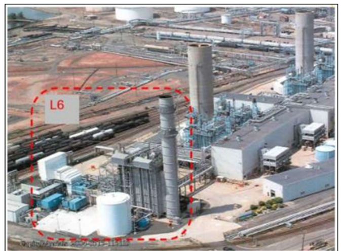
Figure 17: FlameSheet™ combustion system installation on a 7FA heavy duty gas turbine at Linden Cogen Facility in Linden NJ
