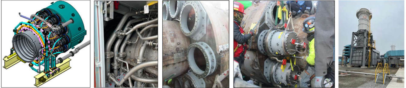
Figure 14: 7EA FlameSheet™ installation at Daesan Korea for high H2 application
