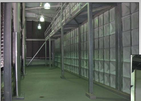
"Unique" pre-filtration system for GTG inlet air, GTG enclosure ventilation and building ventilation
