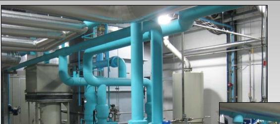
Water cooled generator and lube oil coolers via on-campus chilled water district cooling system
