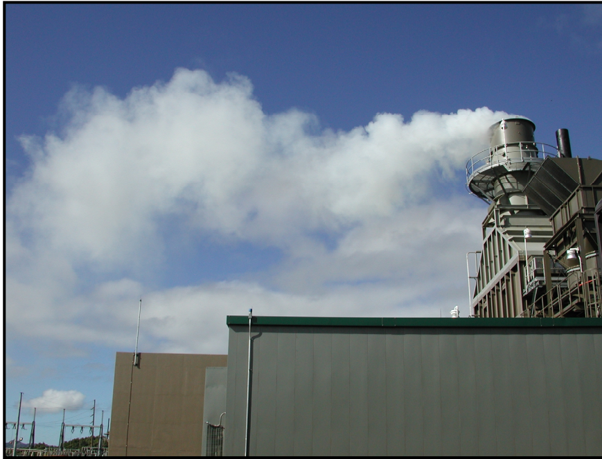
Figure #14 – Exhaust Stack of an OTSG During Soot Cleaning
