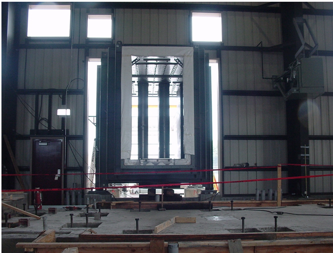
Figure #20 – Inlet Duct Silencer Splitters
