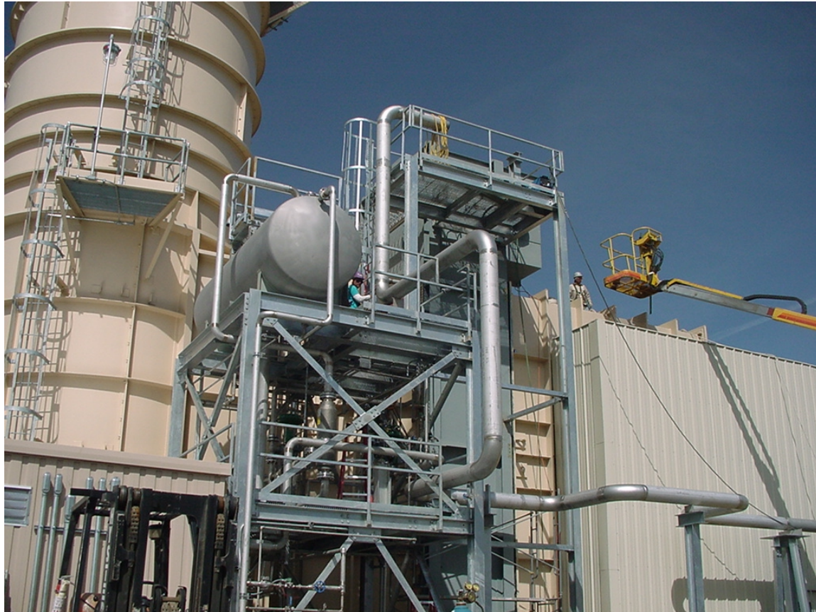
Figure #23 - Acoustic Shroud placed outside of duct walls
