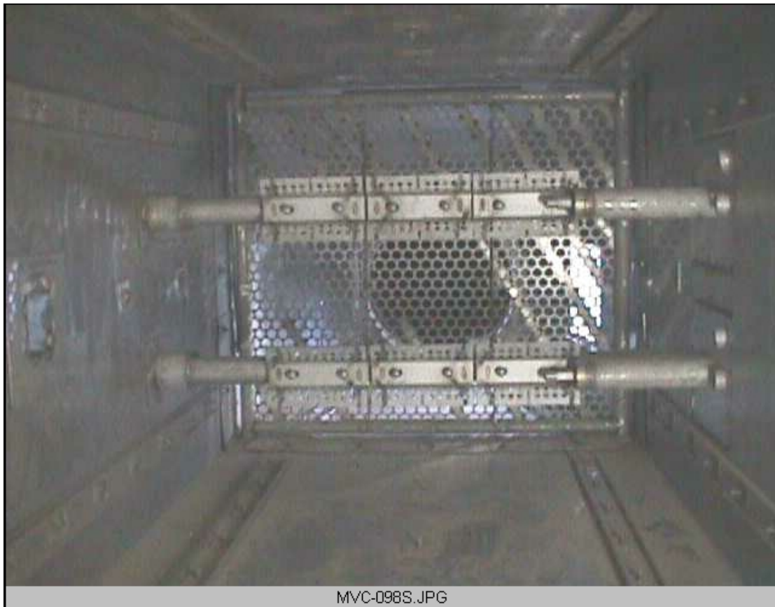
Figure #28 – Variable Porosity Plate
