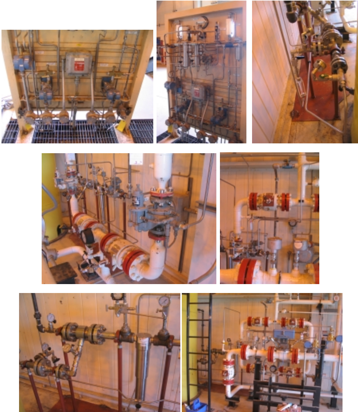
Figure 13: Photos of the Two-Stage Supersonic Ejector Skid Connected to the Fuel Gas System at a 24 MW Gas Turbine Unit.
