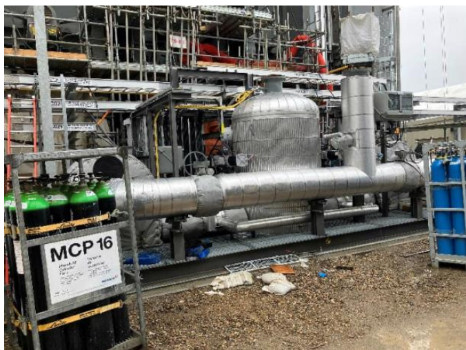
Figure 16 – SCR System at Cascade
