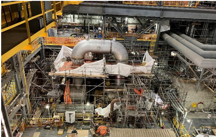
Figure 12 - ST Crossover Pipe Installation at Cascade
