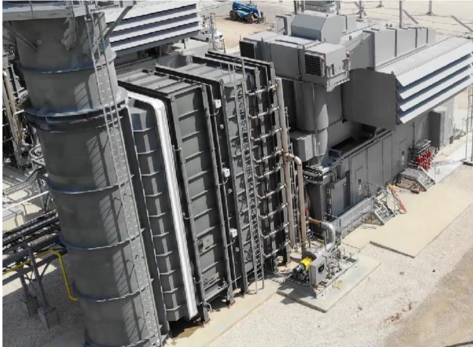
Figure 2: Typical SCR/CO Emissions Control System Behind an LM6000.
