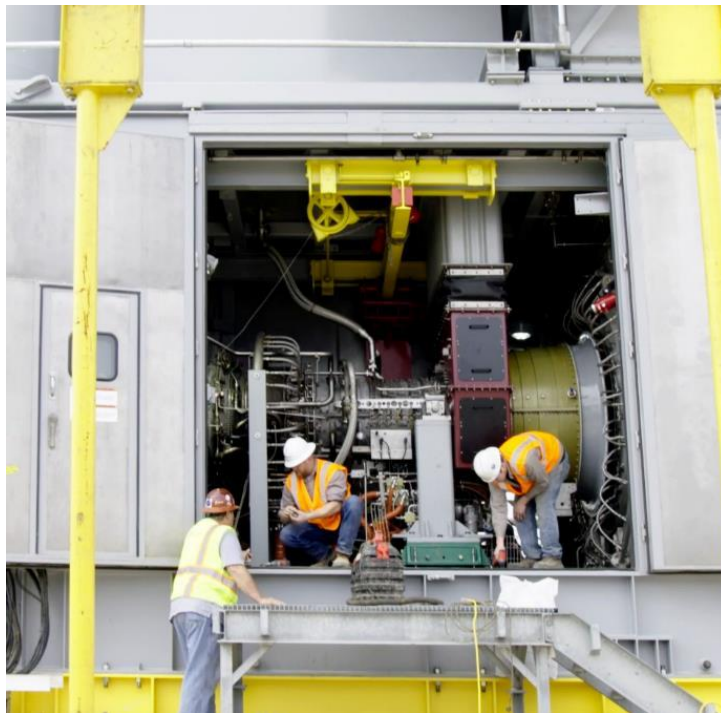
Figure 7: LM6000 Turbine Access Doors.
