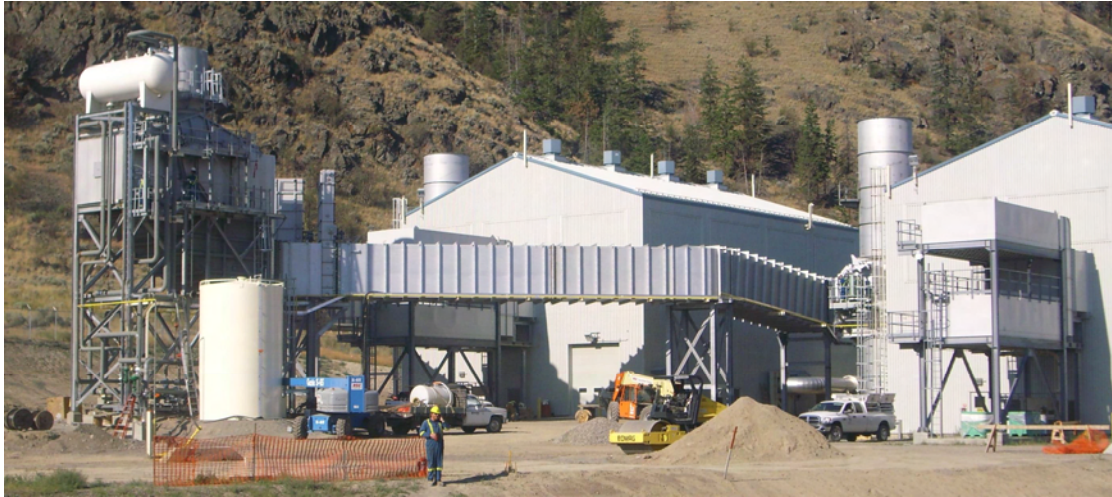
Figure 4 - Photograph of the Savona Exhaust Handling System
