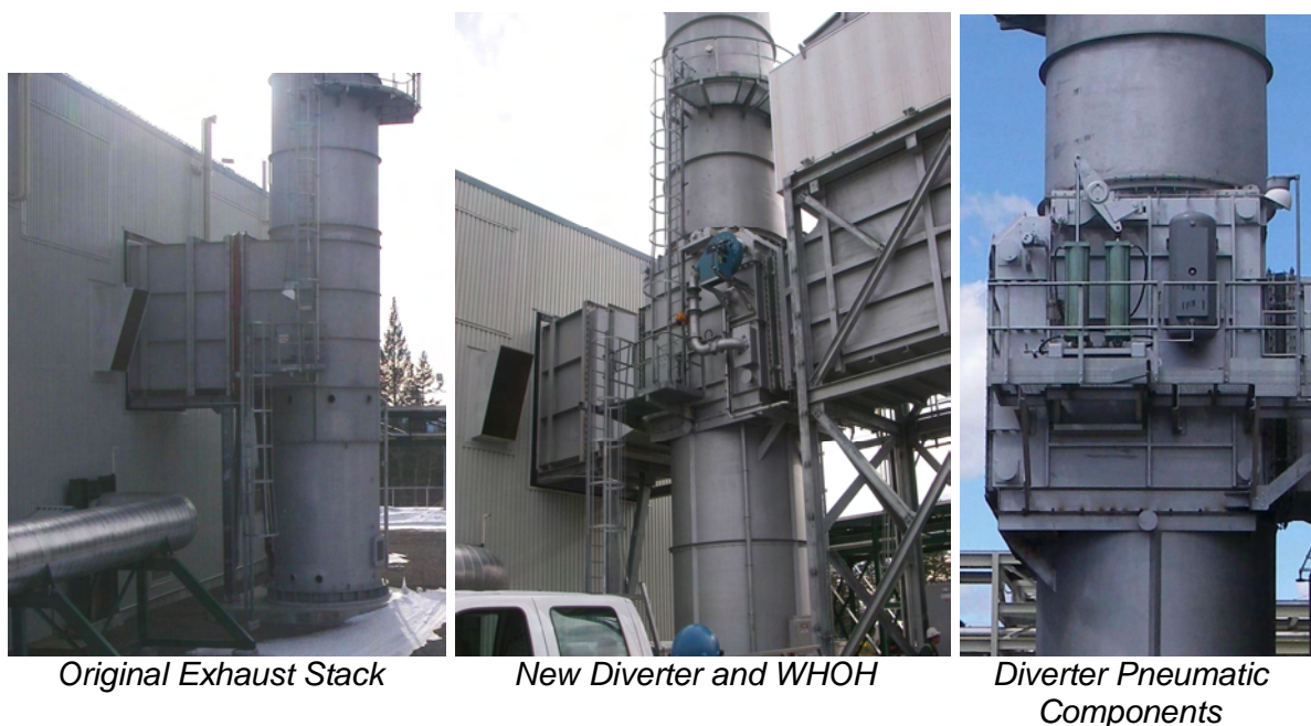
Figure 3 - Photographs of the 150 Mile House Diverter Installation
