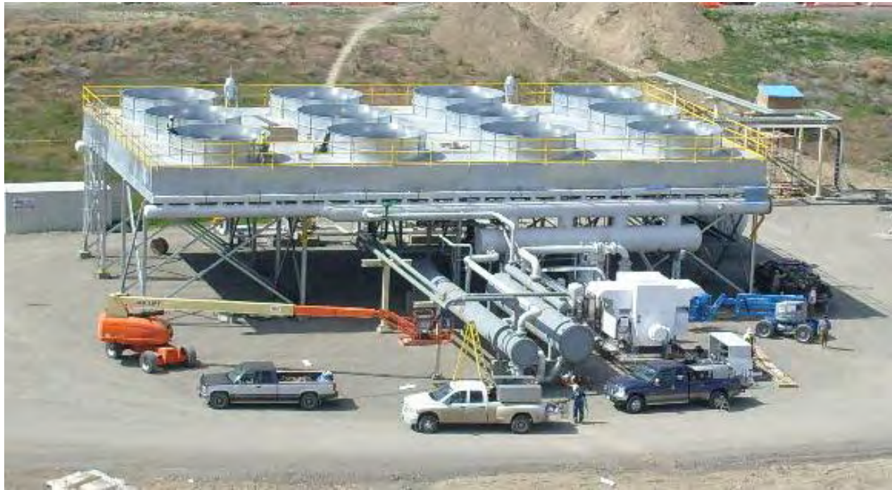
Figure 7 - Photograph of the Savona ORC System
