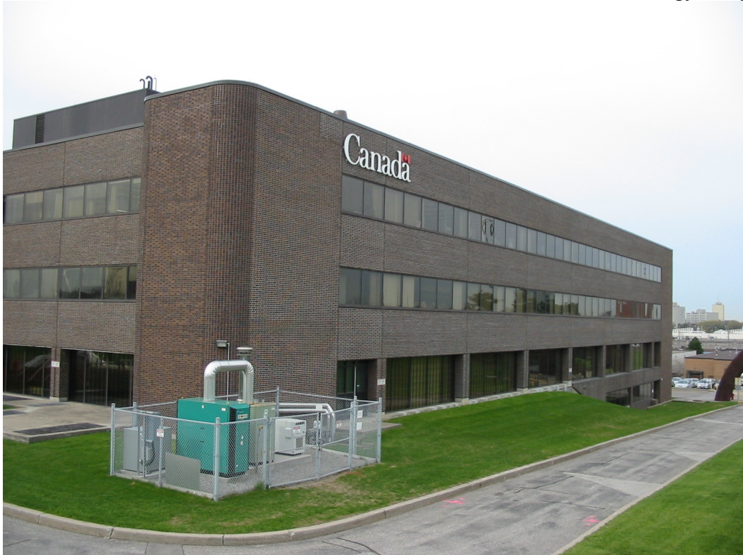
Figure 2 Cummins 60 kWe with Unifin heat recovery unit, Health Canada, Toronto
