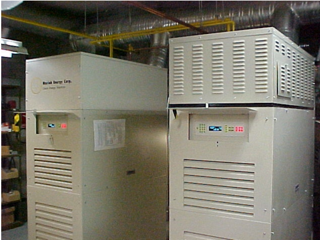
Figure 1 Two Mariah 30 kWe/60 kWt. Southern Alberta Institute of Technology, Calgary
