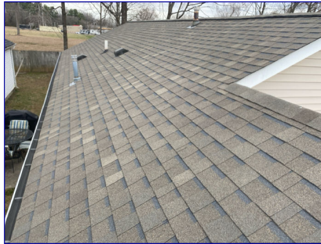
The Roof View
