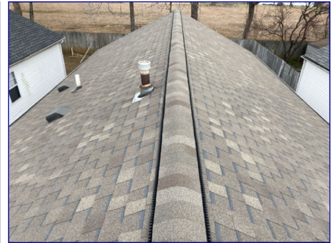
The Roof View
