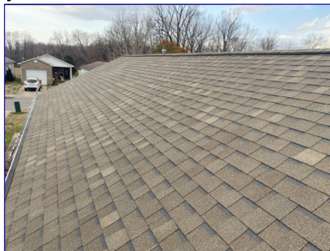
The Roof View
