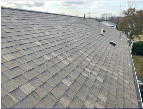
The Roof View
