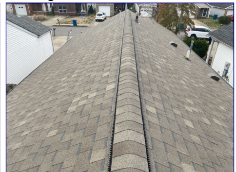
The Roof View
