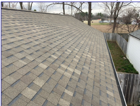
The Roof View
