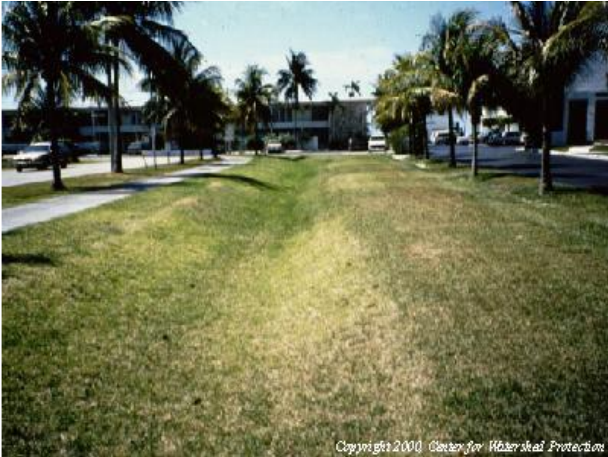
Above: dry swale for filtration;
