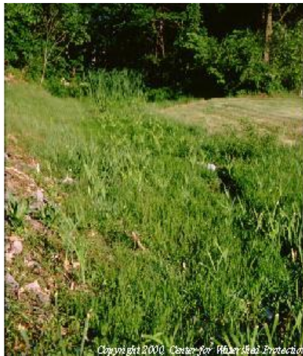
Above: dry swale for filtration;
