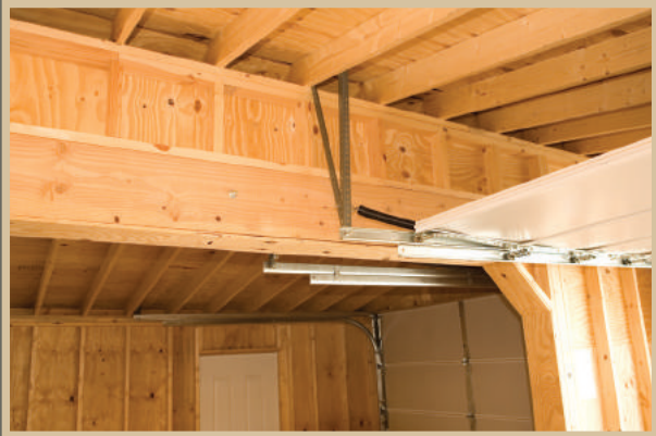
Modular section detail showing central beam & connecting construction.
