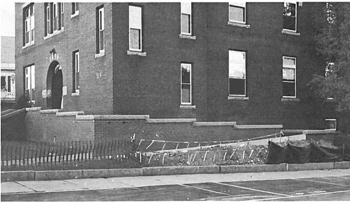
The progress on the Town Hall front entryway continues to move forward. The front steps are in place, as are the upper and lower ramps. At the time of photo what remains to be done is the finishing concrete to be poured.
