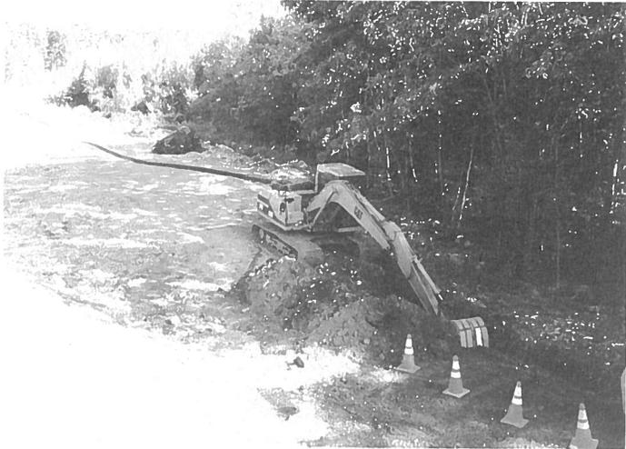
Equipment of the Alton Water Department is seen here at work last month as a new six-inch water main is buried under the "back access" road to Jones' Field. The main is to connect the town's third well with the existing water distribution system at River Lake West Street. The 500 g.p.m. well was driven last autumn, and when the connection is placed in service by the end of this year, the town's water supply will be more than doubled.
