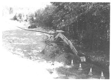
Equipment of the Alton Water Department is seen here at work last month as a new six-inch water main is buried under the "back access" road to Jones' Field. The main is to connect the town's third well with the existing water distribution system at River Lake West Street. The 500 g.p.m. well was driven last autumn, and when the connection is placed in service by the end of this year, the town's water supply will be more than doubled.
