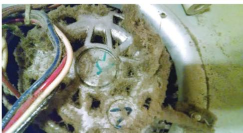
A dirty, inefficient blower caused by air bypass from a 1" filter.
